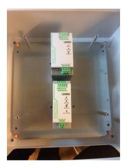
Reinstall middle plate. Remember the earth connections under one of the bolts.
